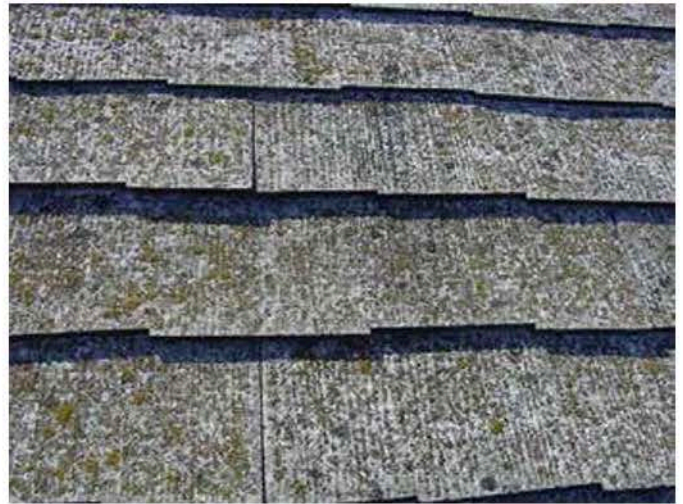
Transite Roofing Shingles
