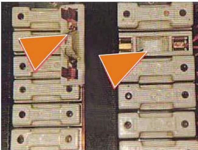
Asbestos Rope (electrical fuse board)
