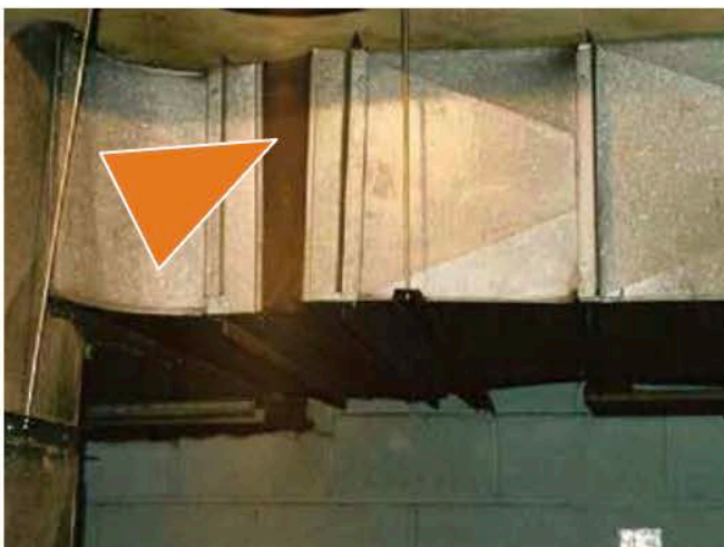
HVAC Vibration Damper (boot fabric)
