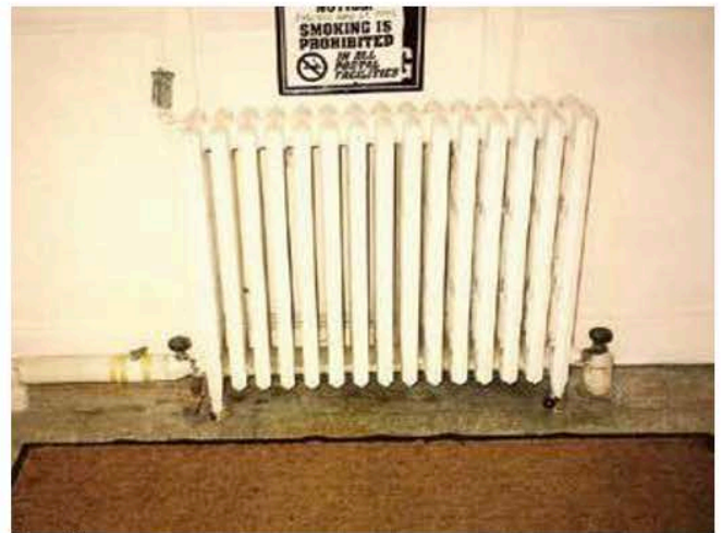
Radiator (insulation on piping and valves)
