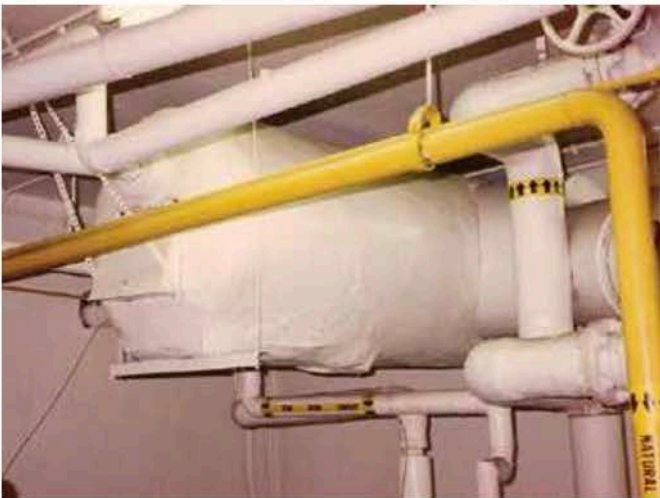
Tank Insulation
