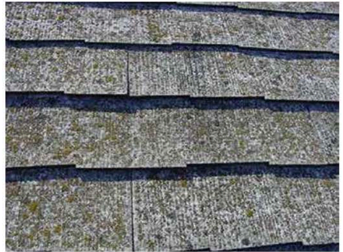
Transite Roofing Shingles
