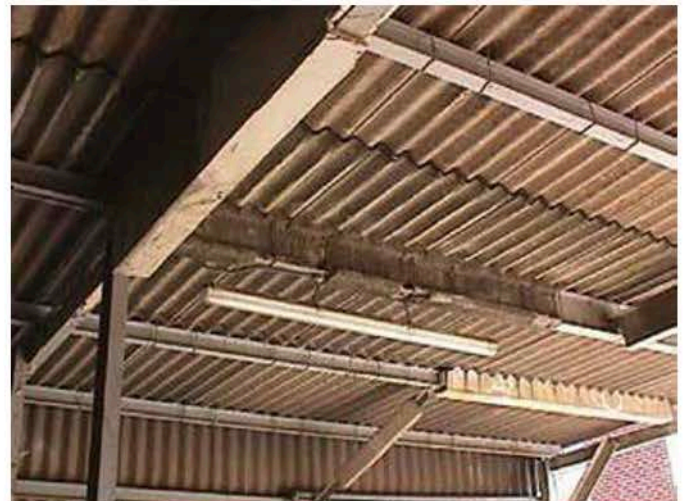
Corrugated Transite Roofing (cement board)
