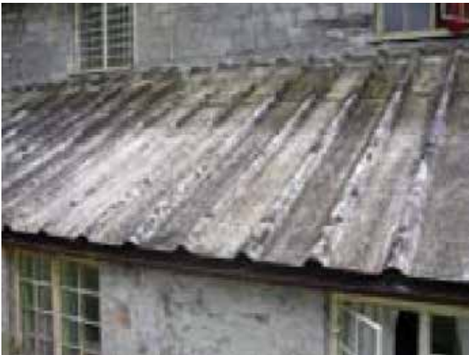
Transite Roofing (cement)
