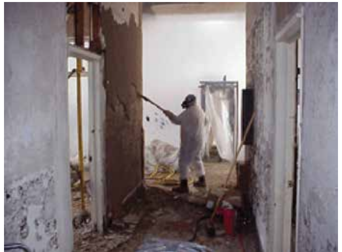
Plaster Walls (being removed)
