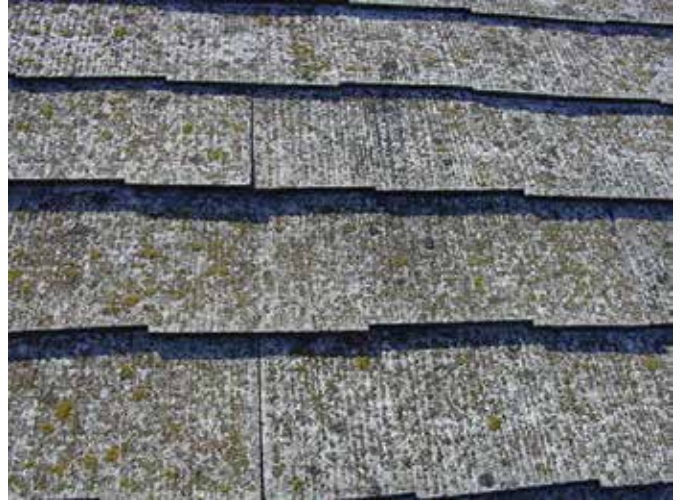
Transite Roofing Shingles
