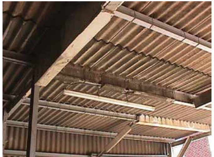
Corrugated Transite Roofing (cement board)
