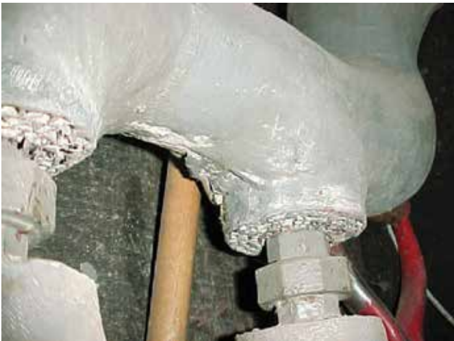
Pipe Fittings (air-cell and mud-plaster type coating)
