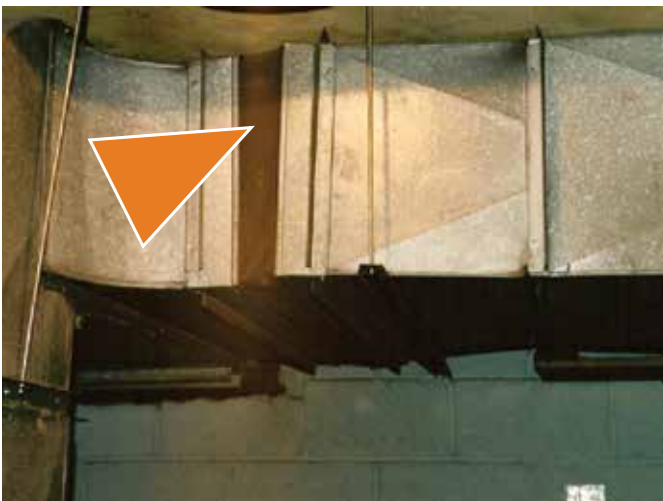
HVAC Vibration Damper (boot fabric)
